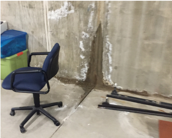
Foundation wall leak in Basement
